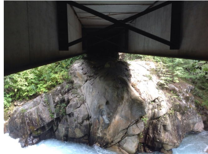
Left Bank Abutment when facing downstream
