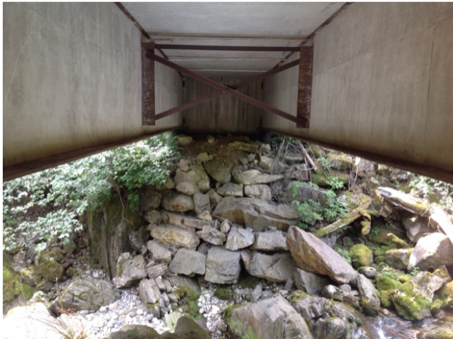
Right Bank Abutment when facing downstream
